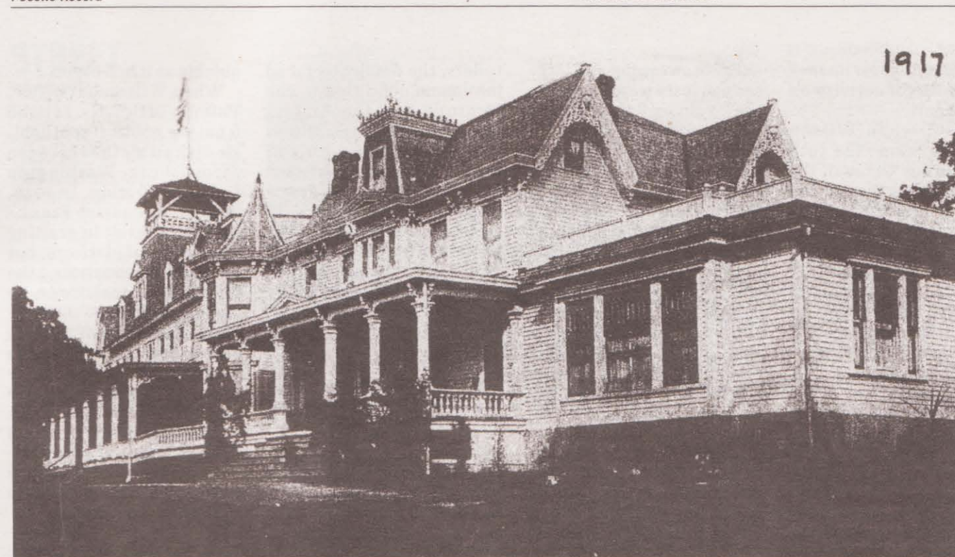
Churleigh Inn, the summer home of the Collinses. Sam Collins had Churleigh Inn built on top of Godfrey Ridge where they lived during the summer months and then in Harriet Hall during the winter. PHOTO PROVIDED
